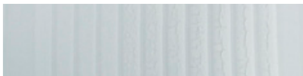
HEC Cracking > 14 Mils (0.36 mm)
